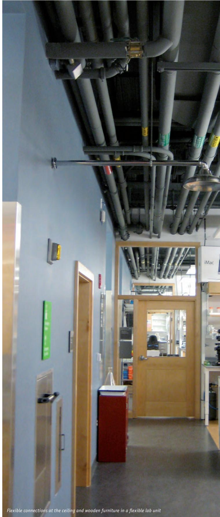
*Flexible connections at the ceiling and wooden furniture in a flexible lab unit*
